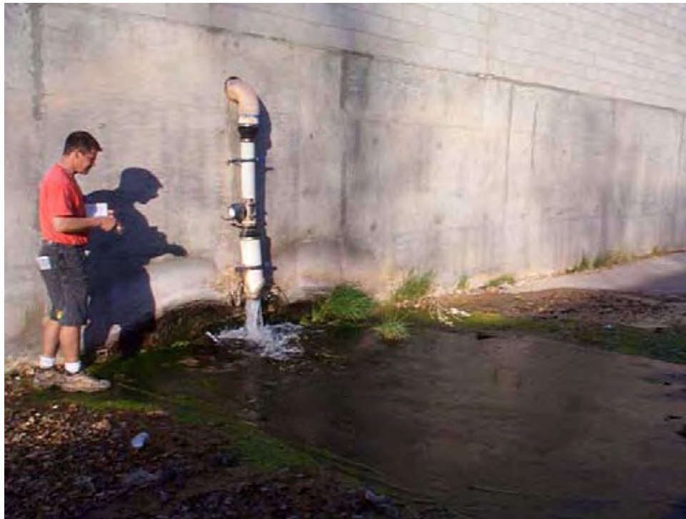
Figure 4. Photo of the Domino Estate dewatering outfall. This outfall functions as the start of perennial flow in Duck Creek.
