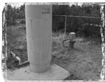
A typical domestic well
