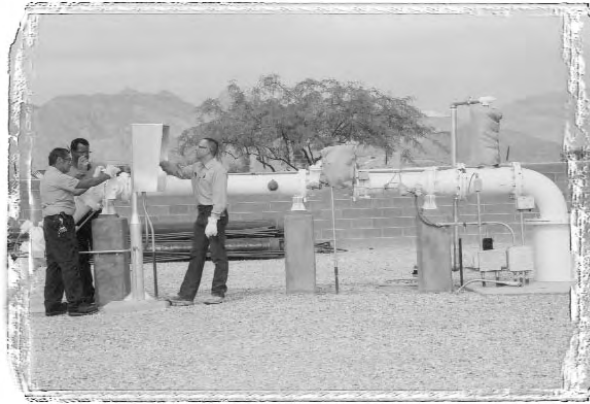
Technicians monitor a recharge well in the northwest valley.
